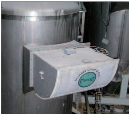
Q-Box application in the food industry with optional sanitary cover: Keeps the Q-Box ③ clean!
