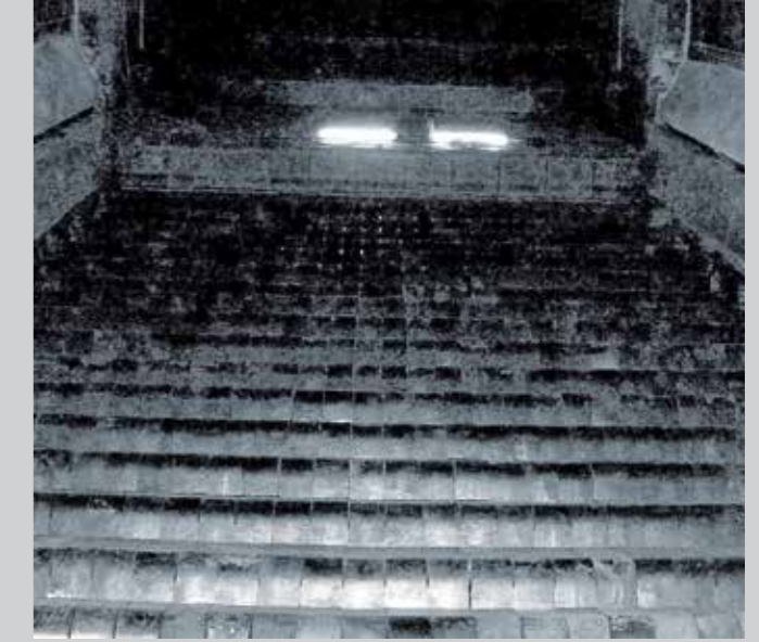
Grate bars in waste incineration
